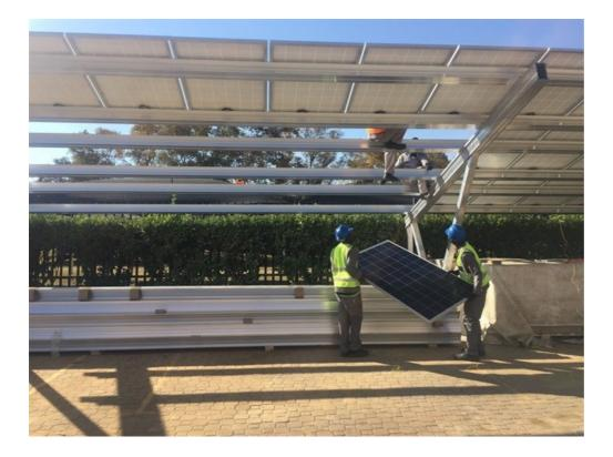
Kevin Norris, consulting solutions architect for Jasco Power & Energy, explains that due to the Westerly orientation of the phase one project, as a result of the existing carport layout, peak solar generation occurred in the early afternoon, matching the peak load profile of the Jasco campus, which occurred as a result of commercial operations and air conditioning loads.
