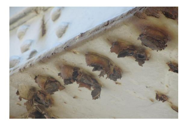
I cannot emphasise enough how vital it is for designers and consulting engineers to specify hot dip galvanised bolts with +60 microns of zinc coating as opposed to electroplated bolts with 12 microns of zinc coating for all South African coastal installations.
