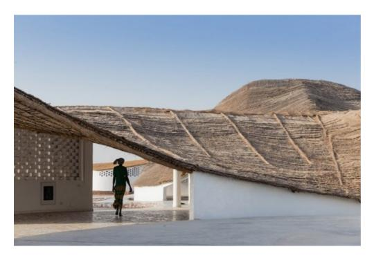
The structure was built from a bamboo framework with fitted rammed earth bricks, which help absorb heat during the day and dissipate warmth at night. The thatch roof is designed to promote rainwater collection, provide shade and promote natural ventilation.
